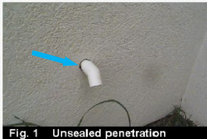
Fig. 1 Unsealed penetration
